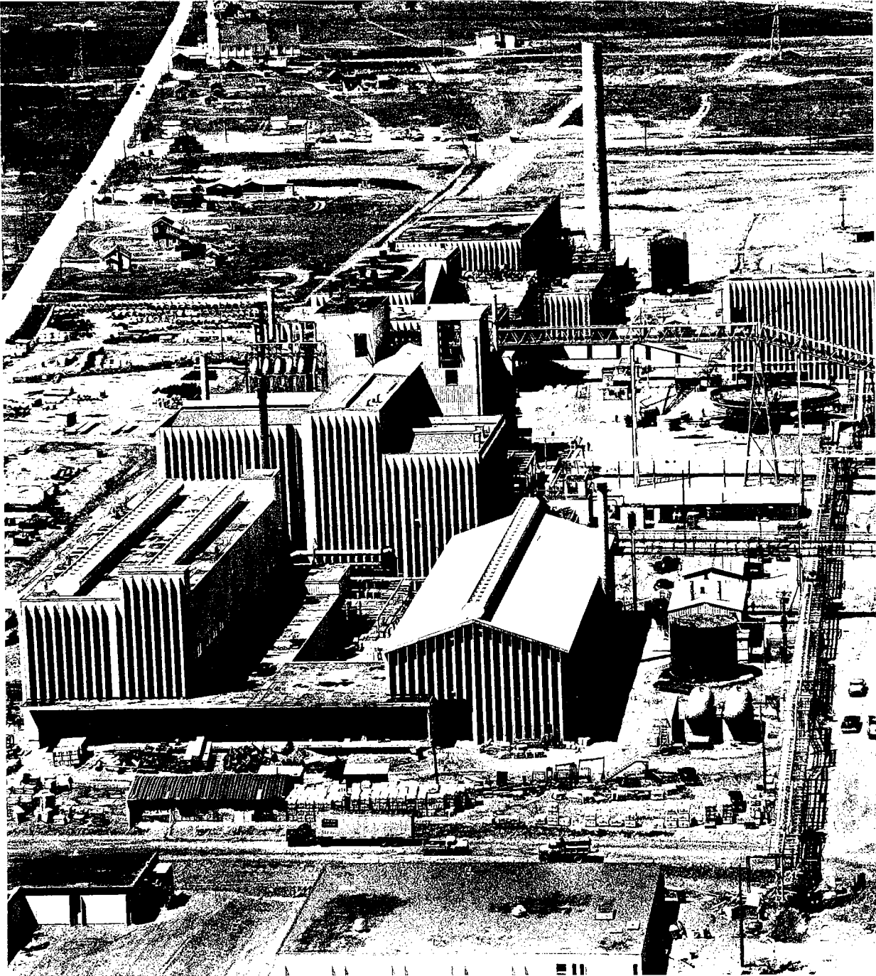
THE CROWNING TOUCH TO NEW BRUNSWICK'S BASE-METAL INDUSTRY: The lead-zinc-silver refinery of East Coast Smelting and Chemical Company Limited at Belledune on Chaleur Bay, nearing completion in 1966.
