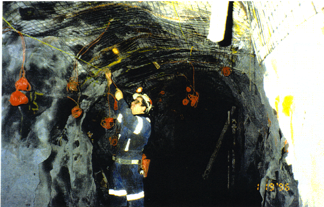
Figure 8a. The drift 3420E before the blast - Section 5 350 E (east view).
