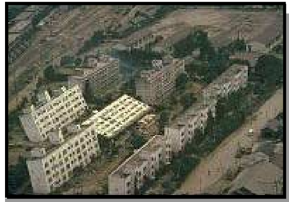
Niigata, Japan, June 16, 1964 Earthquake. Liquefaction undermines otherwise structurally sound buildings.
