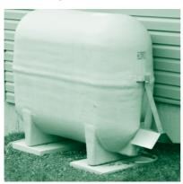
of a newly constructed home. Special attention must be given during these installations to ensure proper stability to support the weight of the tank plus the oil.
