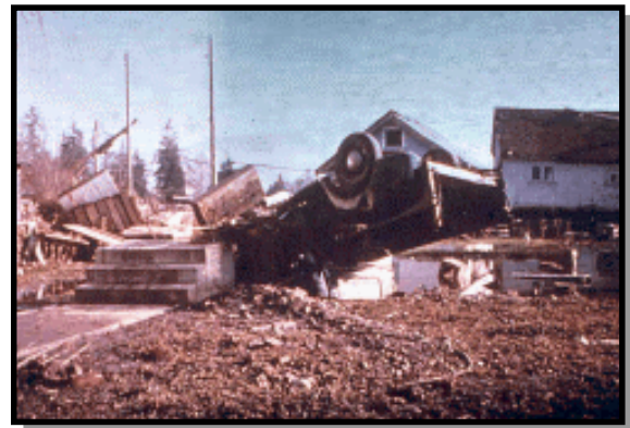
Damage caused by tsunami in Port Alberni, 1964. The power of a tsunami is exemplified as automobile replaces home in this central Vancouver Island community.
