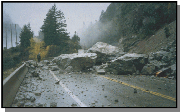
Rockfalls and rockslides are potential secondary impacts of earthquakes. — Provincial Emergency Program, Government of BC
