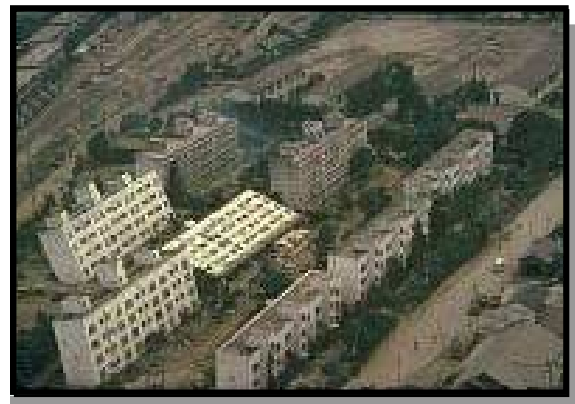
Niigata, Japan, June 16, 1964 Earthquake. Liquefaction undermines otherwise structurally sound buildings. — Earthquake Engineering Research Center, University of California, Berkeley
