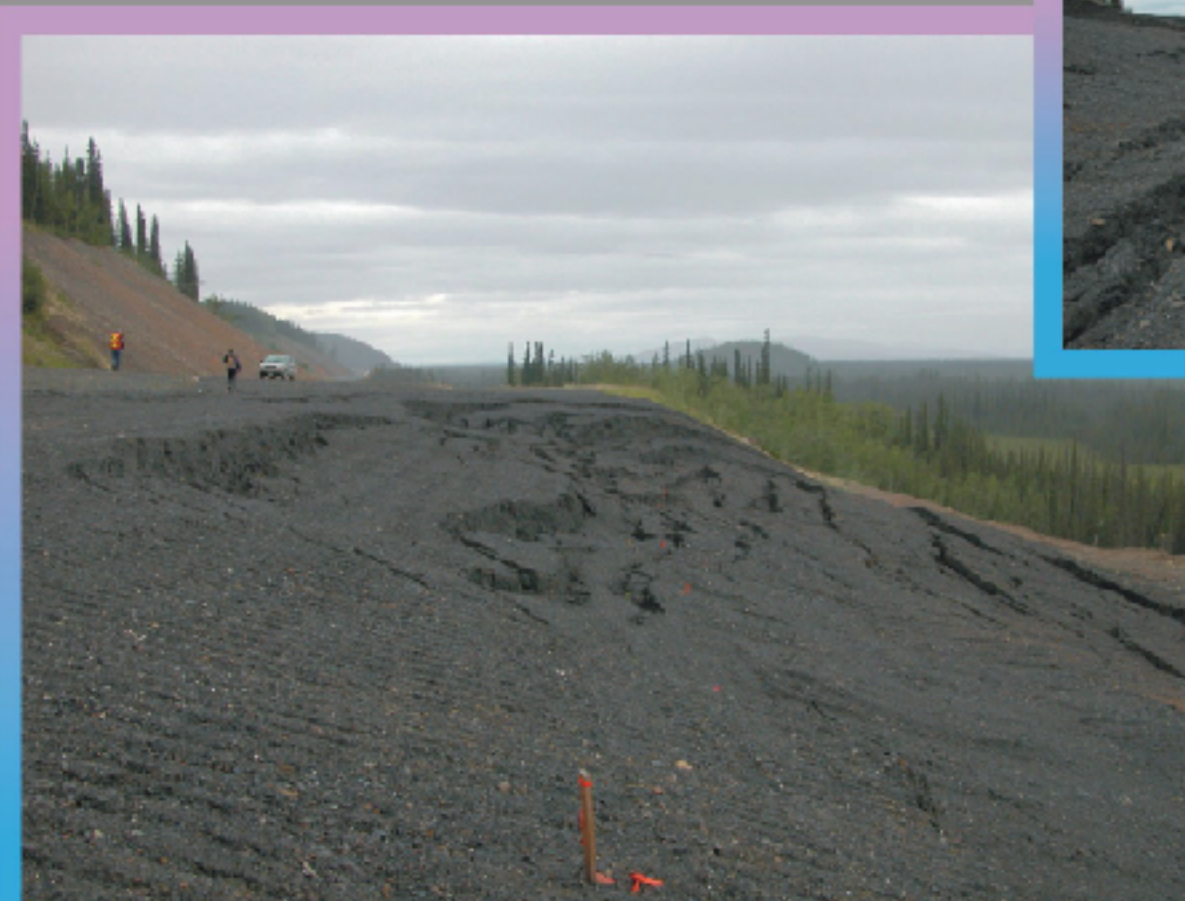
1 Beaver Creek Embankment failure along new highway approach caused by flow of a massive segregated ice lens. This failure formed by groundwater discharge at the base of a bedrock valley wall into permeable glacially derived sands, gravel, and silt. Inset shows magnitude of ground movements.
