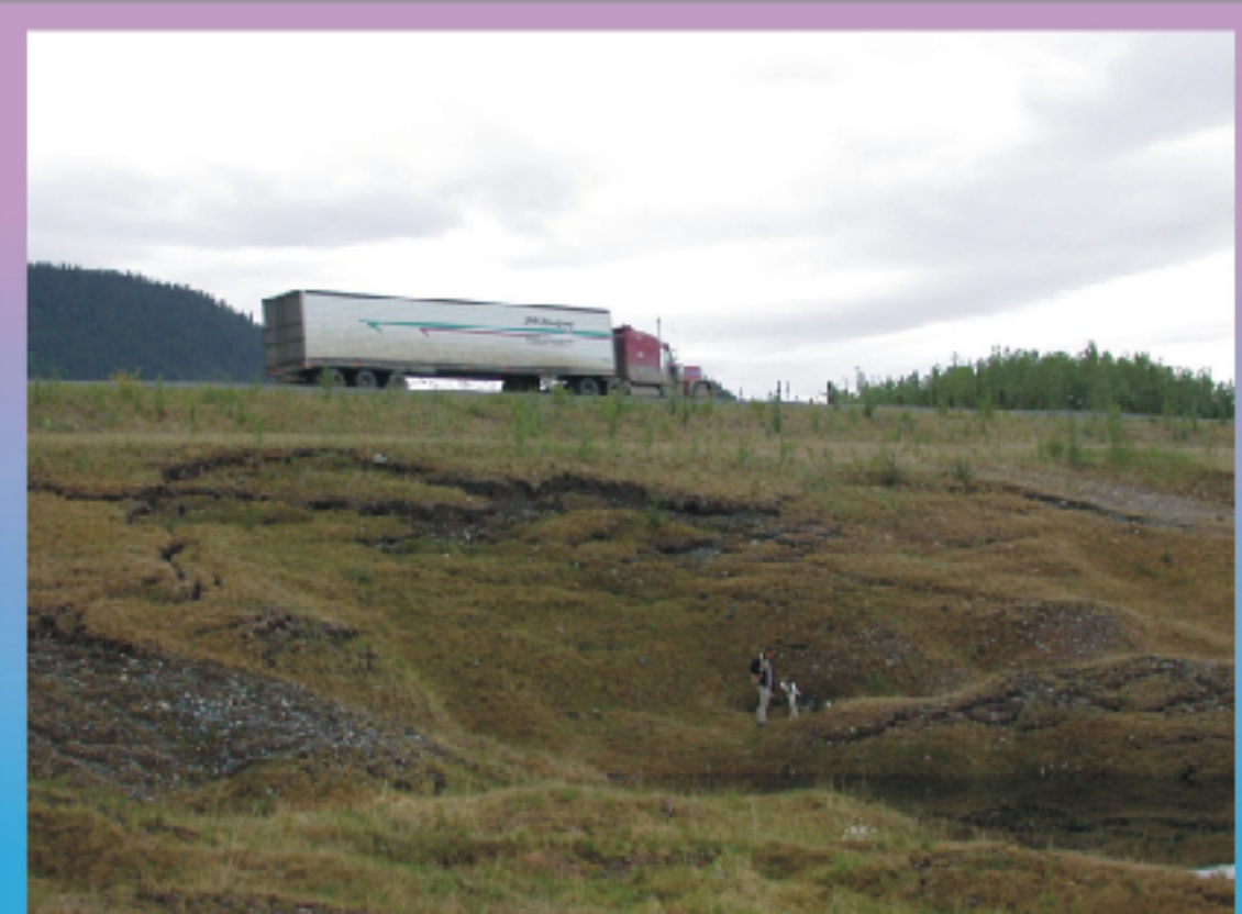
2 Beaver Creek Permafrost subsidence in abandoned gravel pit adjacent to Alaska Highway. Subsidence is related to thermokarsting caused by gravel and vegetation removal adjacent to highway.
