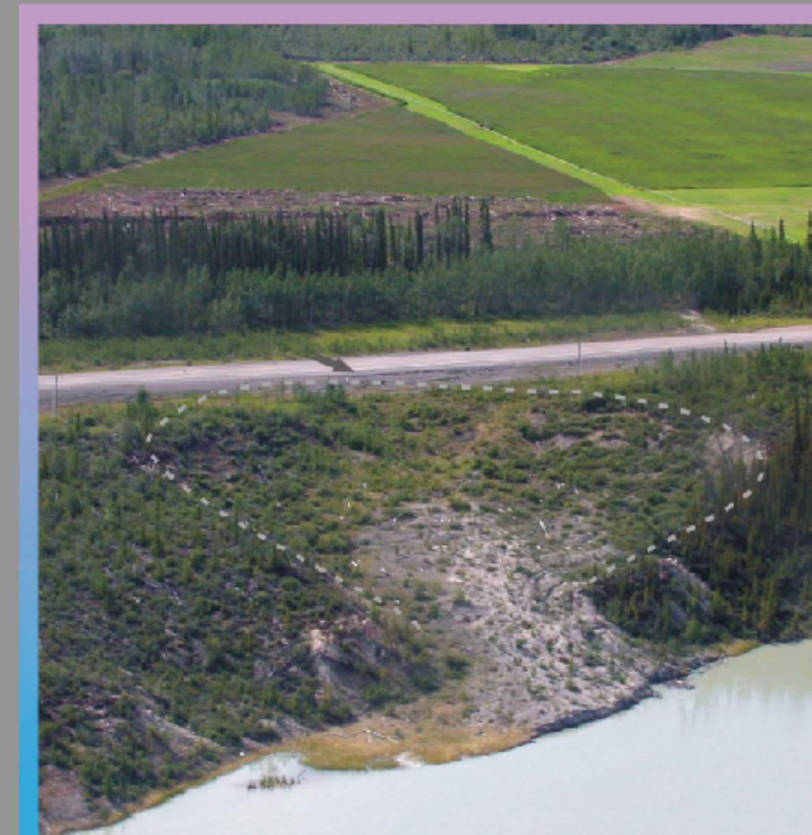
7 Takhini River Abandoned retrogressive ground ice slump in the Takhini River Valley adjacent to Alaska Highway. Note new cracks in highway fill as heeswall stabilizes (arrow). Permafrost thaw related to river undercutting, forest fire, proximity to highway, and forest cover removal in adjacent agricultural fields may contribute to permafrost degradation and the failure. Dashed line highlights remnant roadcarp.
