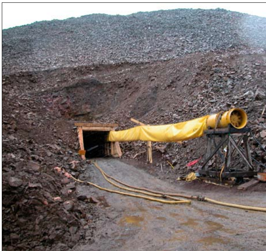
Figure 21. Rehabilitated portal at the MacTung tungsten deposit.
