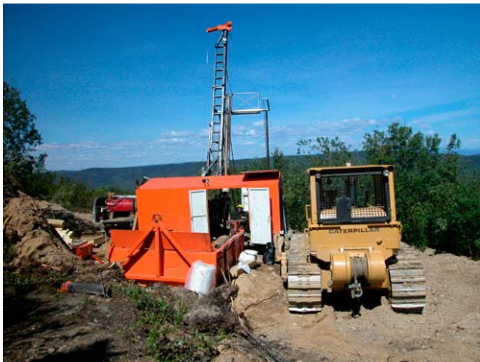
Figure 27. Diamond drill on the Lone Star property.
