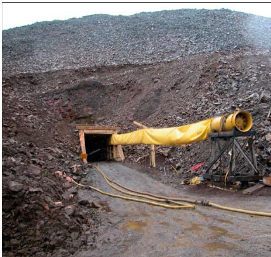
Figure 21. Rehabilitated portal at the MacTung tungsten deposit.
