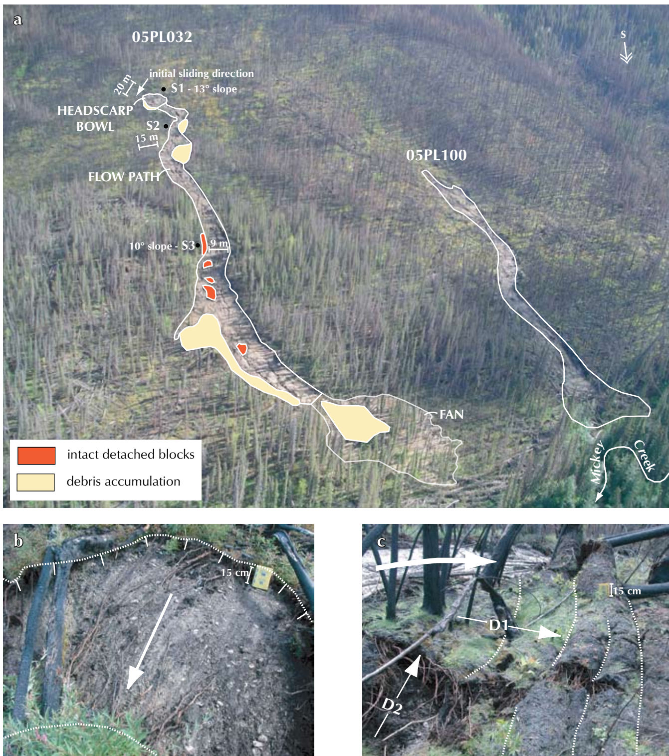
Figure 6. (a) Oblique aerial view of two detachments (05PL032 and 05PL100) that occurred on a gentle south- to southwest-facing slope. The larger failure is over 200 m long and initiated only a few days prior to these photos being taken on July 20, 2005. (b) Detachment of organic mat exposed in tension cracks above the headscarp (location S1 in Figure 6a). Roots are stretched in the direction of sliding. (c) Deformed organic mat (location S3 in Figure 6a), marginal to flow path (heavy arrow). The mat was initially compressed (direction D1) to form folded compression ridges (small dotted lines). It was then torn away from the surrounding mat (direction D2).
