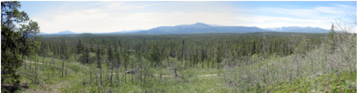
View from the hill above the 138kv transmission line looking south
