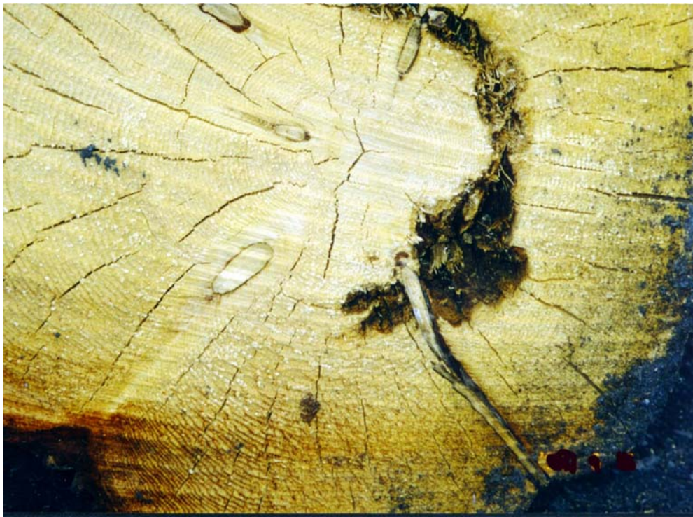
Figure 5.3 Ring rot encompassing approximately 50% of the circumference
