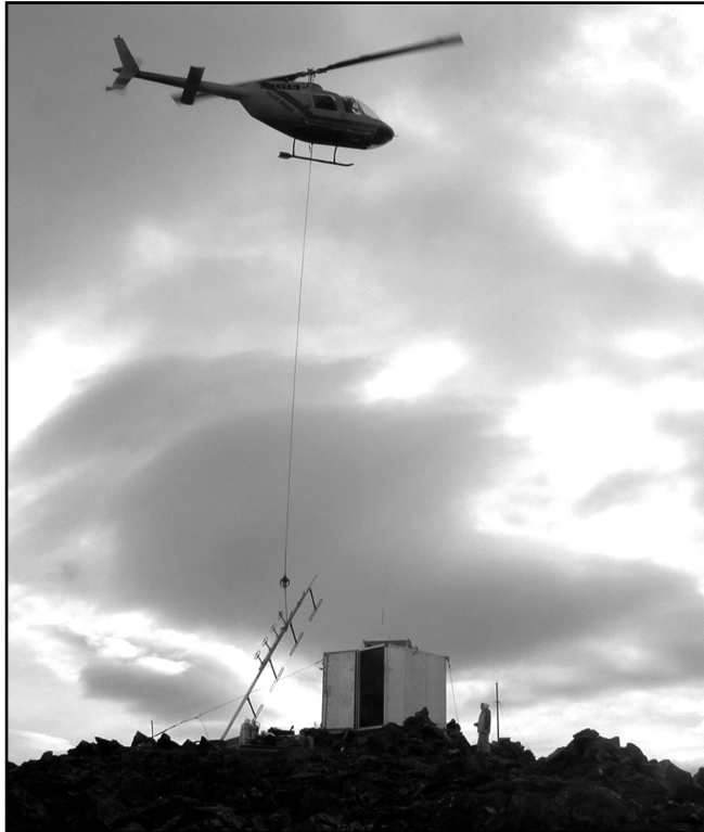
A Bell 206 helicopter airlifts YARA's antenna into position at the Mount Decoeli radio site in August 2002.
