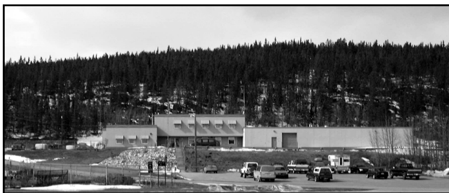
Headquarters of YTG Protective Services
