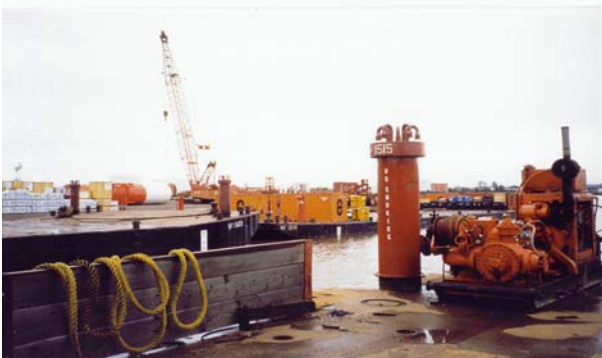
Hay River Barge Terminal
