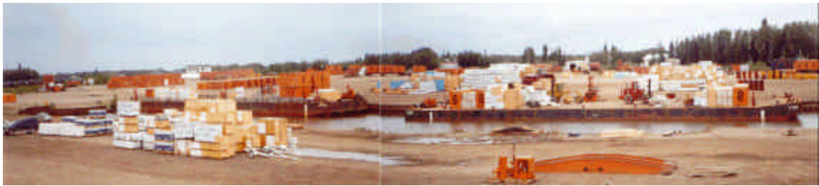
Hay River Barge Terminal
