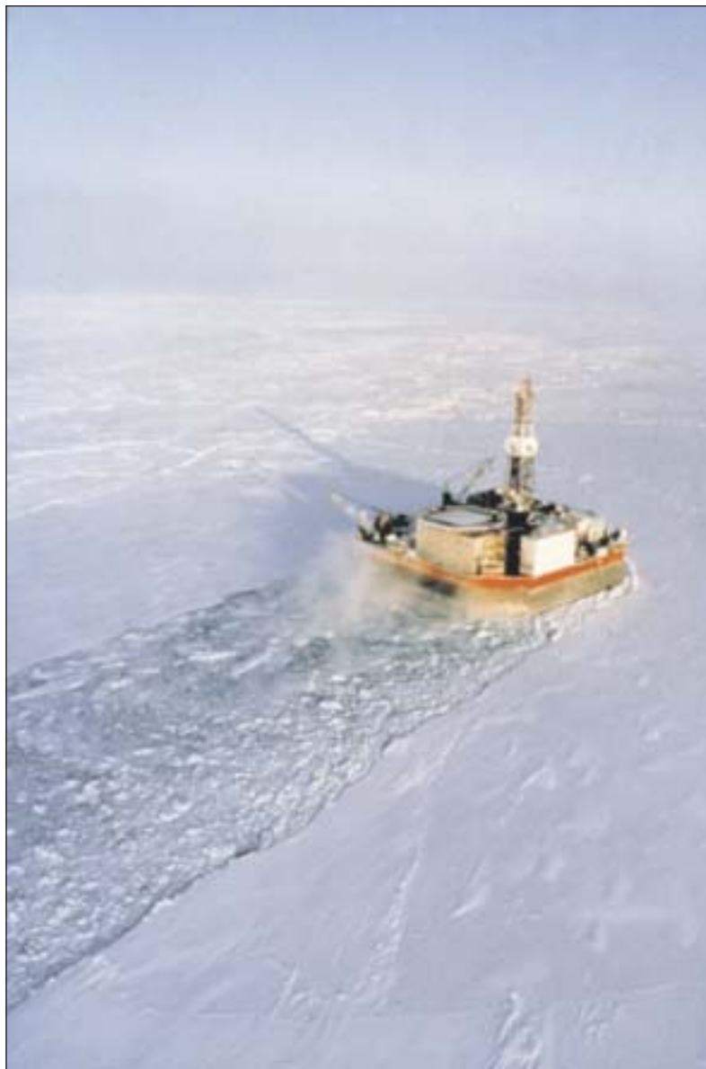
Transition ice pack moving past the Molikpaq drilling caisson, winter ice conditions, Beaufort Sea.
