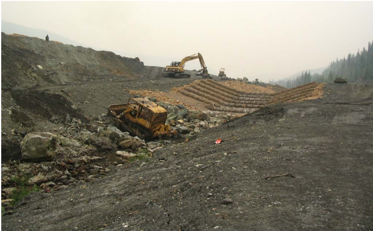
Figure 13 Channel Bed Preparation
