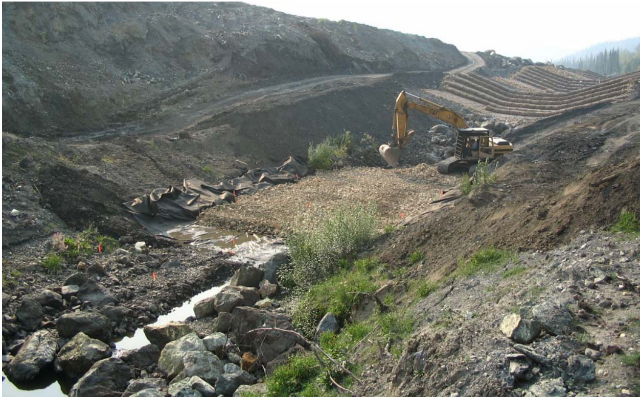
Figure 15 Granular Blanket Drain
