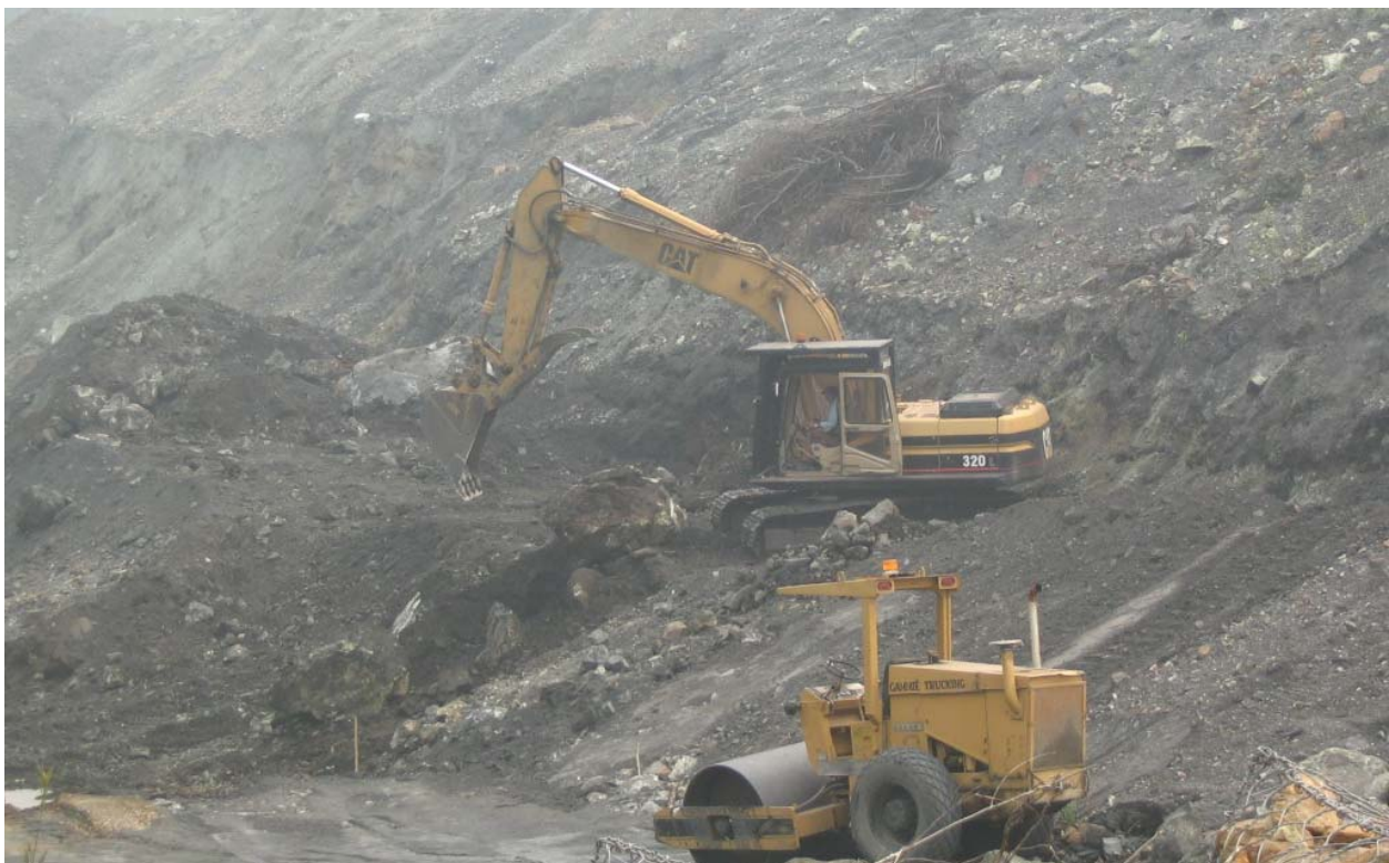
Figure 14 Initial Side Slope Preparation
