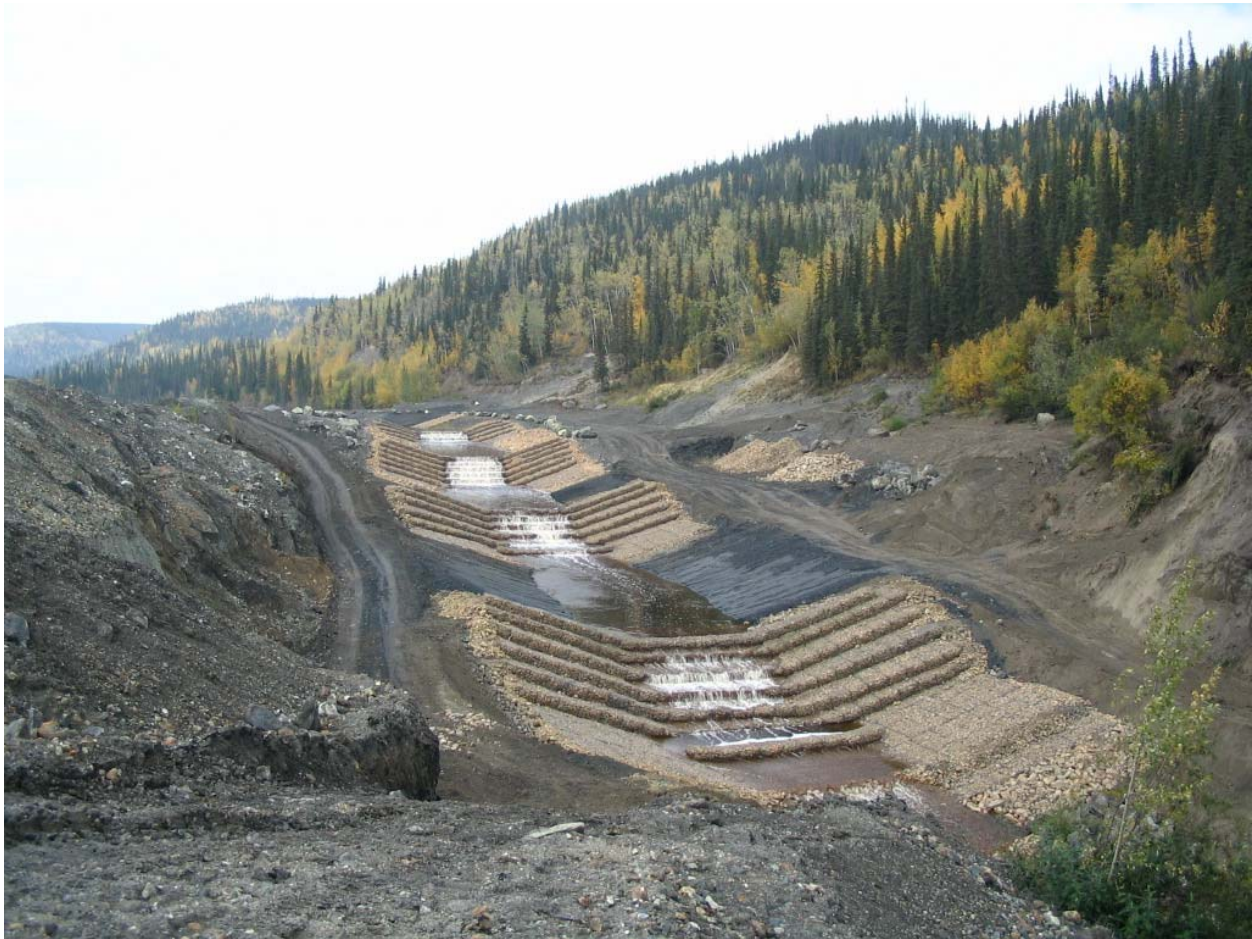
Figure 17 Completed Channel Stabilization Works
