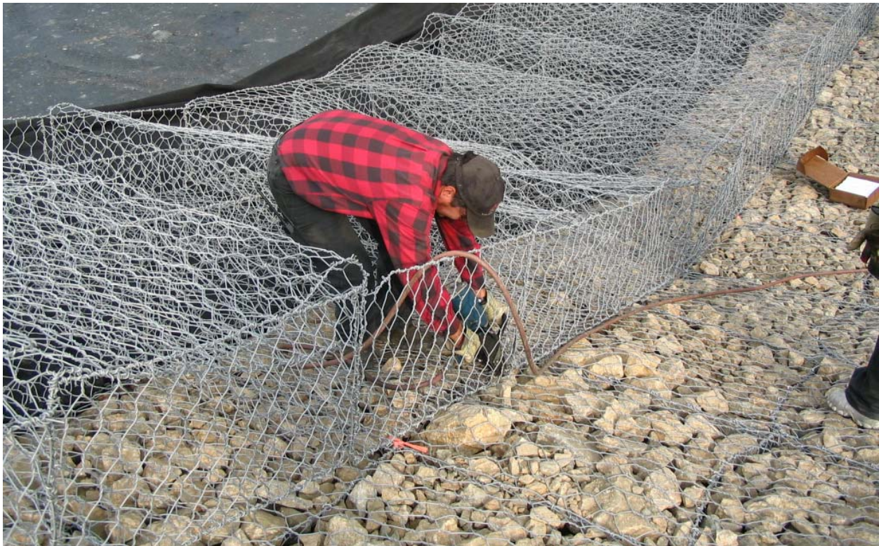
Figure 15 Installing Gabion Baskets
