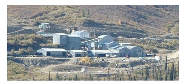
**d) Buildings**: the mill and other buildings could be a safety hazard to people visiting the site. The buildings need to be demolished and the site returned to a more natural state. It is possible that there is contaminated soil around the buildings from gas/oil spills. Any contaminated soil that is found will be cleaned up.
