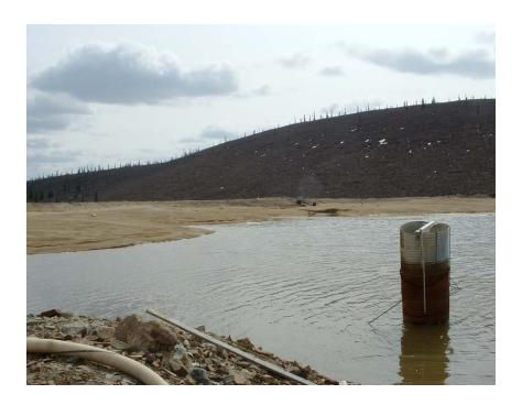
**b) Tailings Dam:** The long term stability of the dam is a concern. The dam was built on permafrost that is beginning to thaw. If there is a very large flood or earthquake, it could break and tailings would flow down the valley. The fine sand could possibly kill fish and destroy fish habitat.
