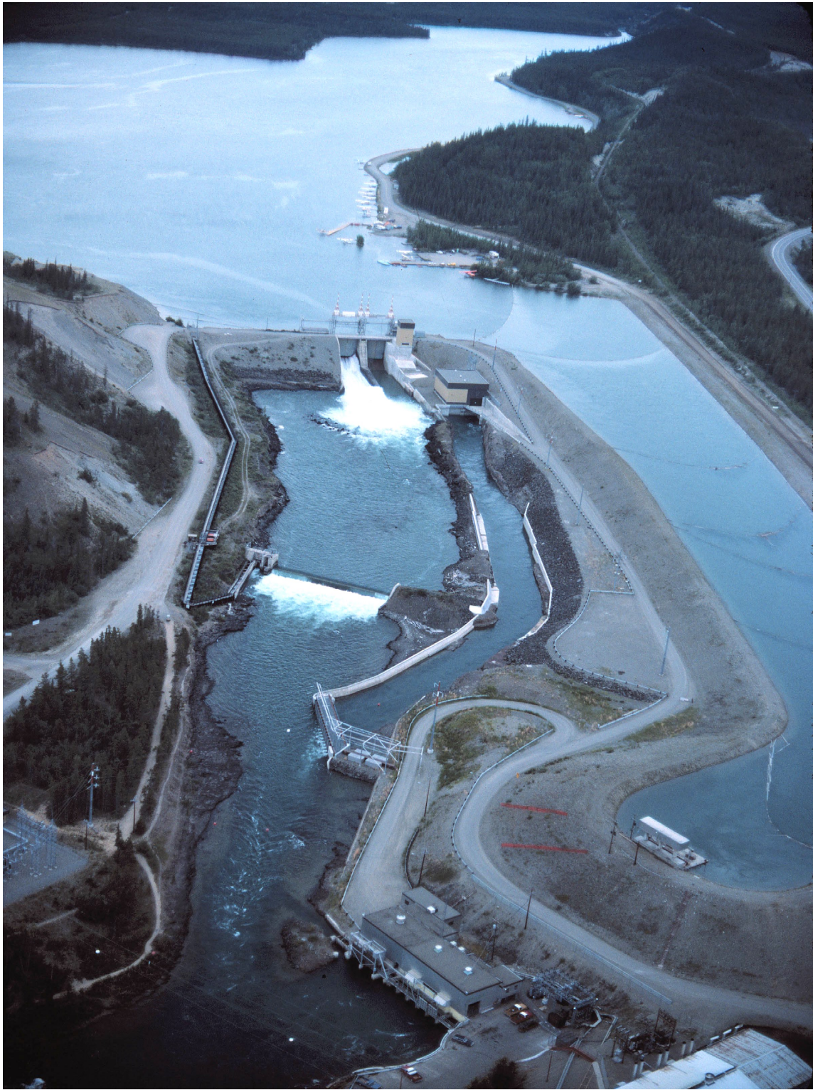
Plate 7. Whitehorse Rapids Hydro Generating Station on the Yukon River (Photograph Courtesy of Yukon Energy Corporation) Pla7
