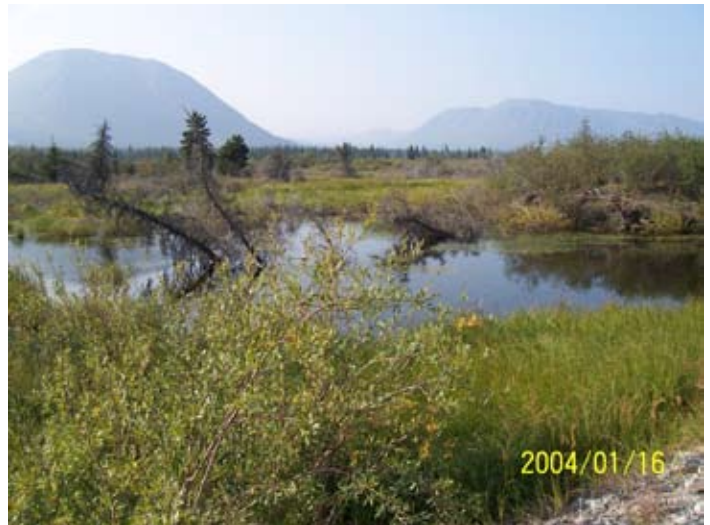
Flooding resulting from road construction.
