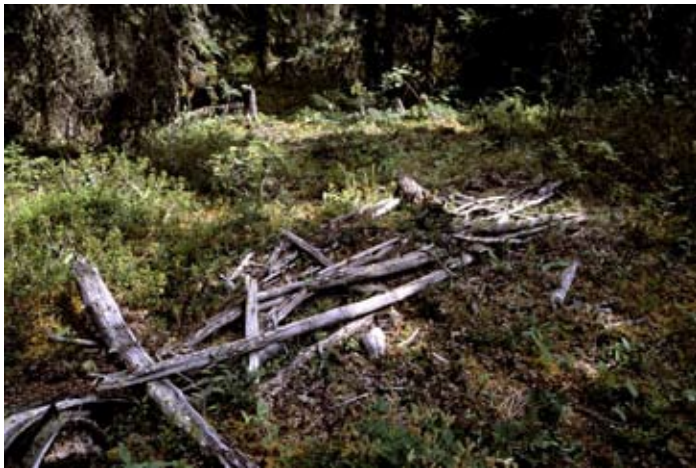
Stage cache collapsed
