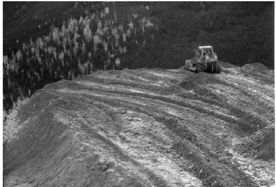
Blading tailings with good soil matrix - likely to revegetate naturally.
