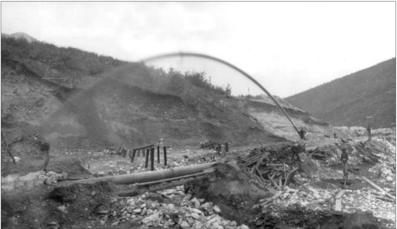
Hydraulic mining operations of the Pacific Coast Mining Co. on Cheechako Hill. (PC, A Johns YT-223)
