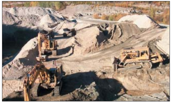
Overview of John Alton and Marty Knutson's mining cut near Grand Forks, showing two excavators digging pay gravel to load into dump trucks, plus one bulldozer stripping waste gravel.
