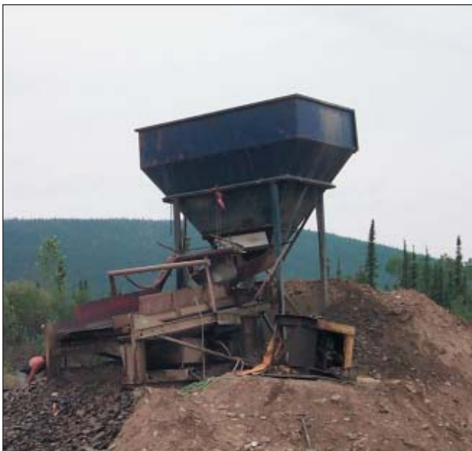
Jim Conklin's processing plant on the right limit of Dominion Creek upstream from Hunter Creek.
