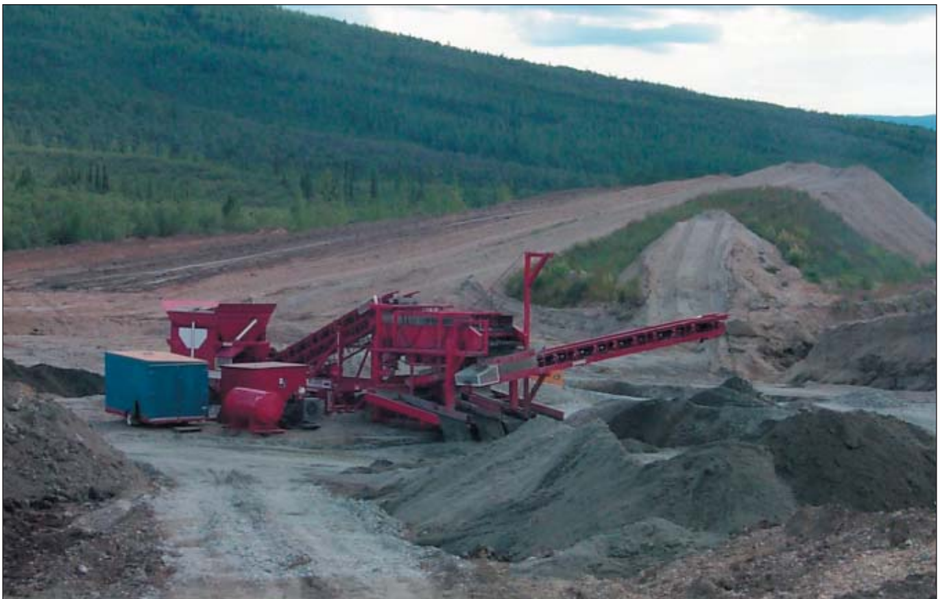
Gatenby Mining Services sluice plant on Dominion Creek.
