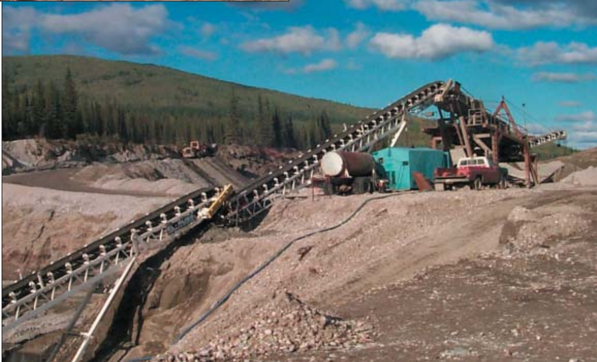
Gimlex conveyors feeding wash plant. (inset) Gimlex relocating fuel tank liner.
