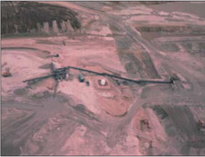
Ross Mining Ltd.'s processing plant on Dominion Creek near Rob Roy Creek in the Dawson Mining District.
