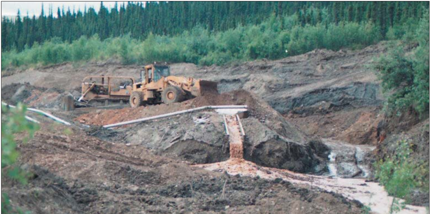
Maurice Alexander’s sluice plant set up on the left limit of the Little Gold Creek valley in 2002.
