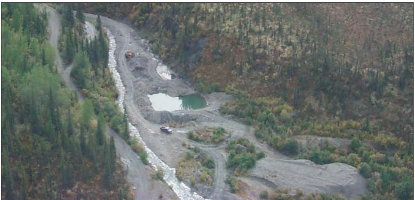
Joe Rabb's Duncan Creek operation in 2001. View looking upstream towards the canyon.
