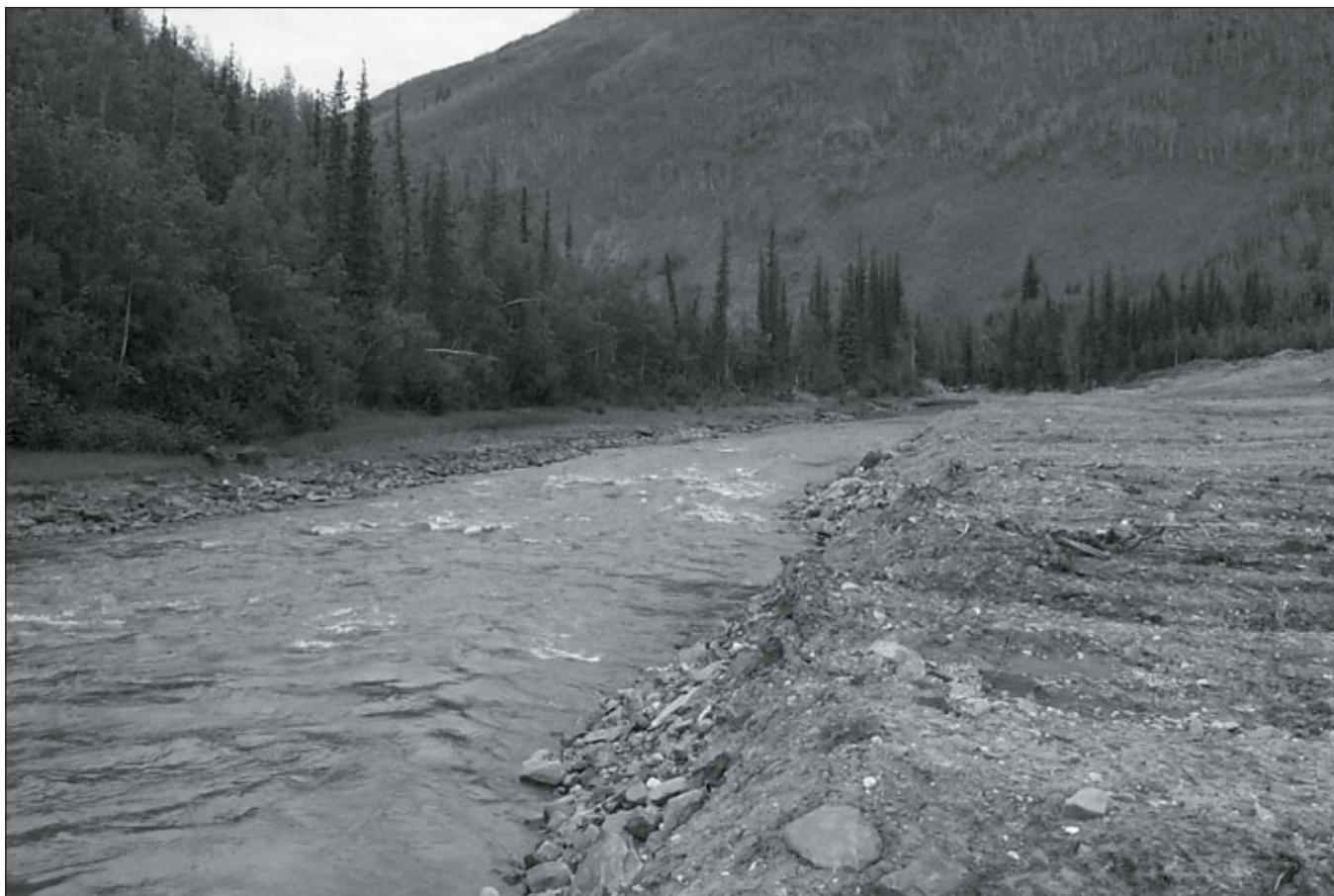
David McBurney's restored river bank, with large rock armouring along the bank and overburden spread up to the edge.
