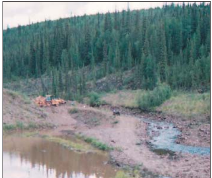
David Cachelin processing a cut on Big Gold Creek in 2002. Settling ponds are in the foreground.
