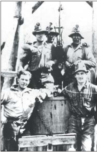
Bucket of Slaves” - Miners in the bucket were lowered into shaft to fill bucket with pay gravels to send to surface. McCormack and Stewart operation, Miller Creek, 1938. From left front, Gus Vinblad, unknown. In the bucket, Jim Lynch, unknown, Johnny Titus.
