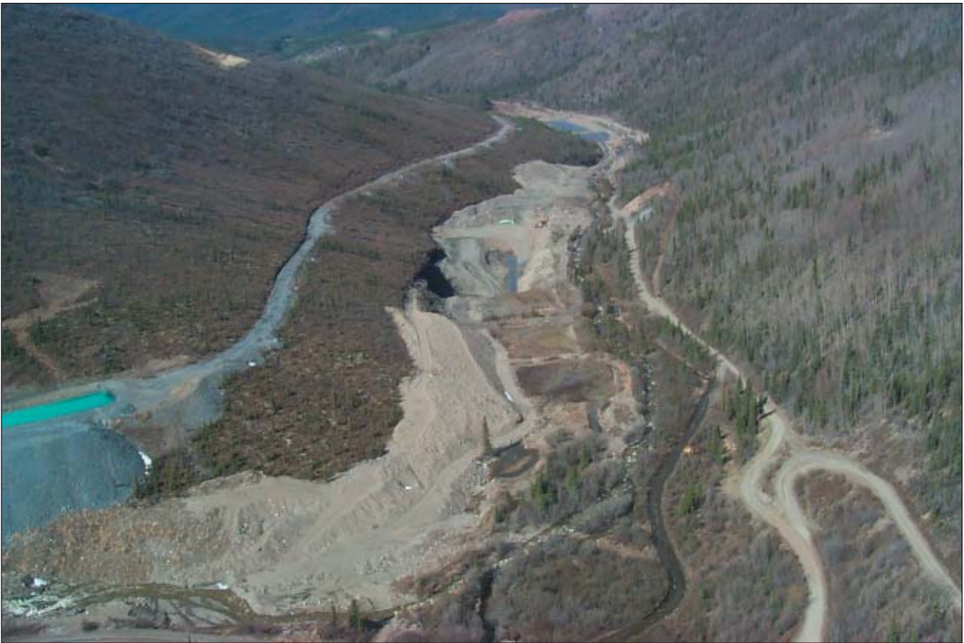
Bardusan Placers' operation on Lightning Creek. View looking downstream.
