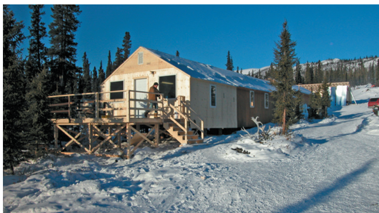
Figure 26. Expanded kitchen facility at the Wolverine camp.
