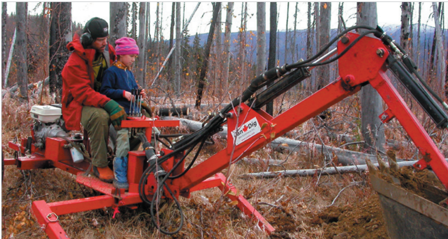
Figure 22. Cheyenne Ryan learning to trench at the White property.
