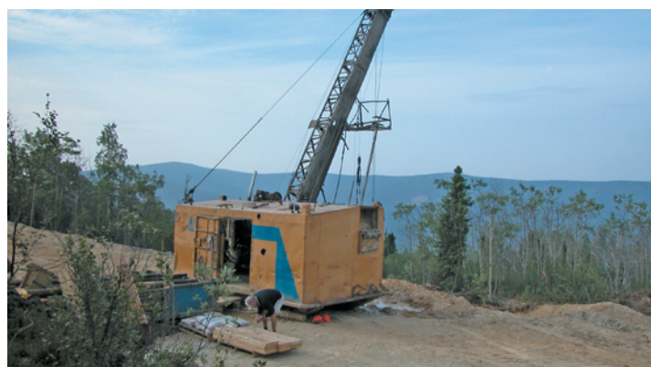
Figure 18. Drill set-up on Klondike Source's Klondike property. The headwaters of Victoria Gulch are in the background.
