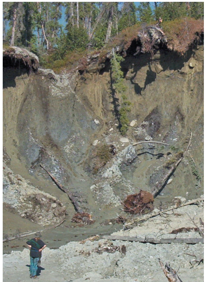
Figure 12. Active scarp, Magundy River landslide, looking northeast.
