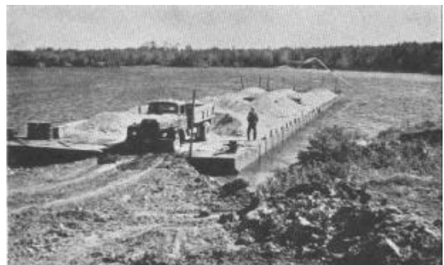
Unloading Gravel Barge at Berens River
