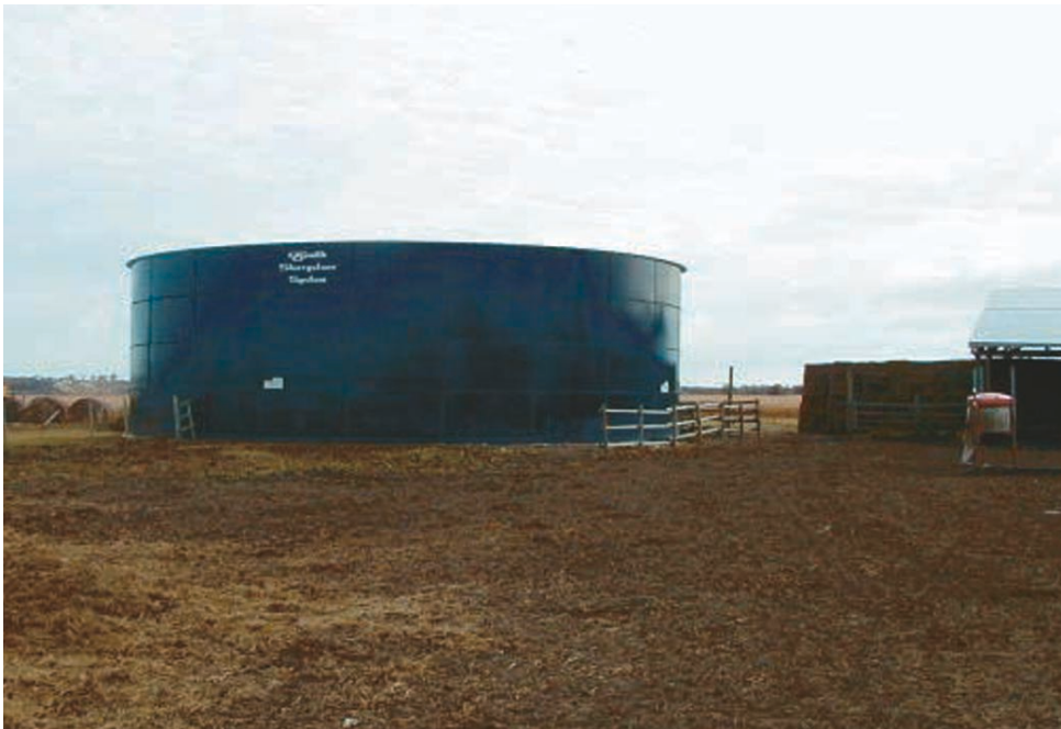
Above-ground steel structure for storage of liquid manure.
