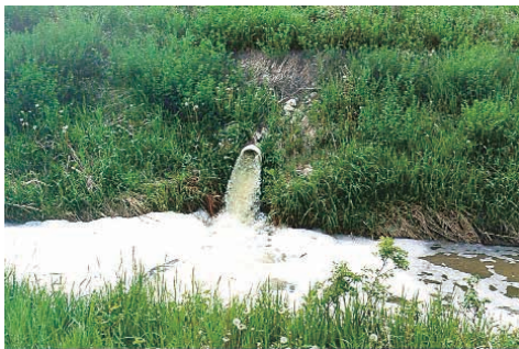
Controllable point source discharge from a municipal lagoon.
