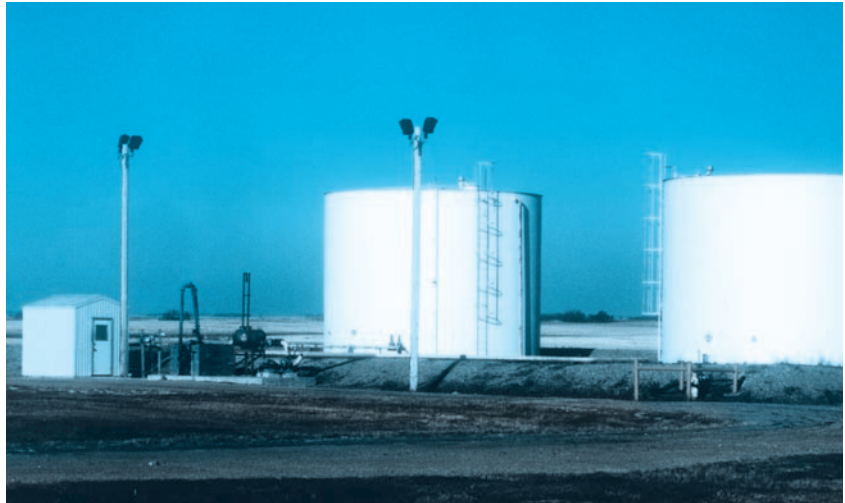
ETHANOL STORAGE TANK
