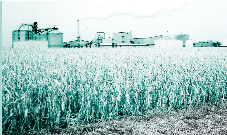
NEW U.S. ETHANOL FACILITY
