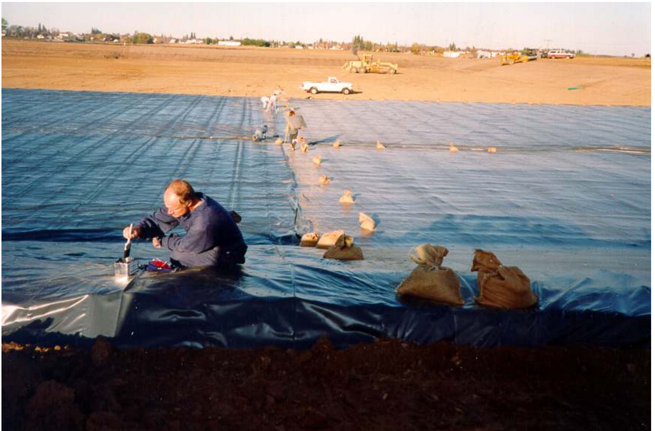
Installation of Synthetic Liner Carberry Lagoon Construction
