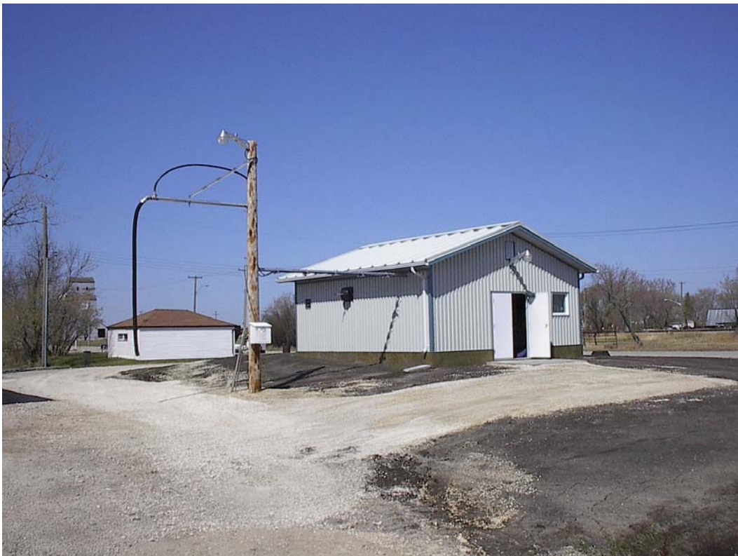
Tank Loading From Reservoir
