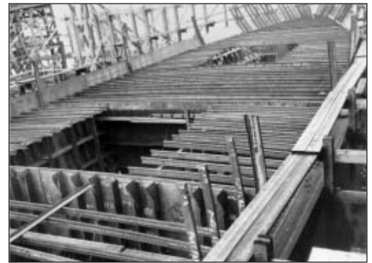
HULL NO. 133 UNDER CONSTRUCTION IN BURREARD DRY DOCK, DECEMBER 1941. (NAC PA187473)
