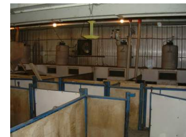
Enclosed Dunging Areas (EDAs) and biofilters shown in the background of one of the rooms.
