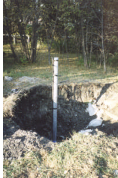
Extension of well casing above grade
