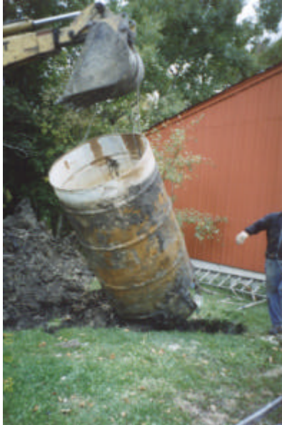
Removal of well pit cribbing
