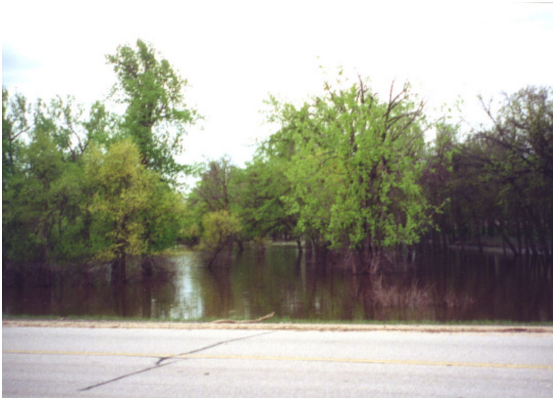
PHOTO E-3: #850 ST. MARYS ROAD LOOKING SW (DOWNSTREAM) FROM NORTHBOUND SHOULDER (May 16, 2001)
