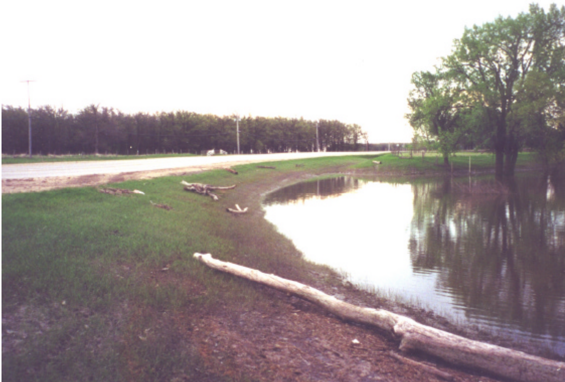
PHOTO E-4: #850 ST. MARYS ROAD LOOKING SE ALONG SOUTHBOUND SHOULDER (May 16, 2001)
