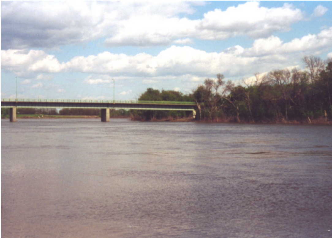
PHOTO E-11: PR #305 BRIDGE LOOKING NORTH AT EAST BANK (May 17, 2001)
