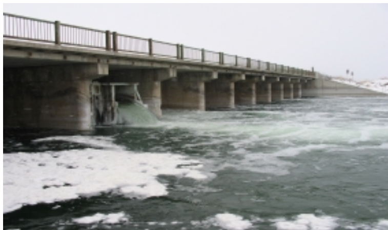
Below: Fairford River Water Control Structure
