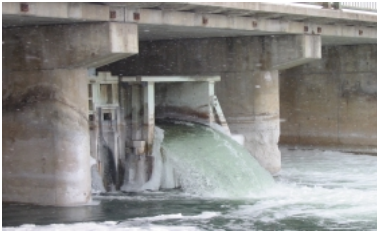
Above: Fairford River Water Control Structure fish ladder, attraction flume.
