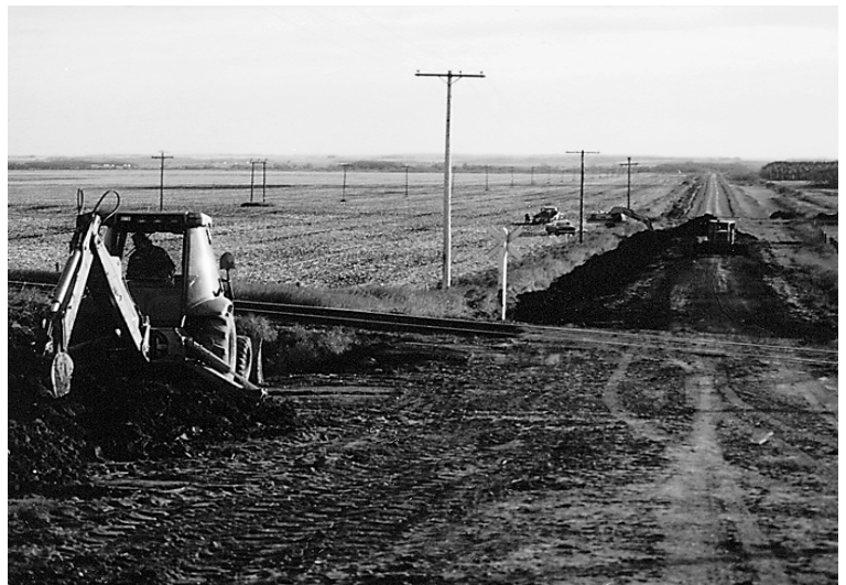
Installing a rural water supply
