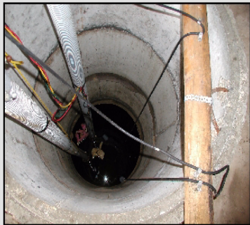
Figure 3: Hulme Tile Outlet Manhole
