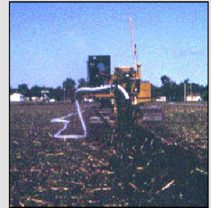
Figure 2: Typical Tile Drainage Installation by Plow (McCutcheon Farm Drainage)
