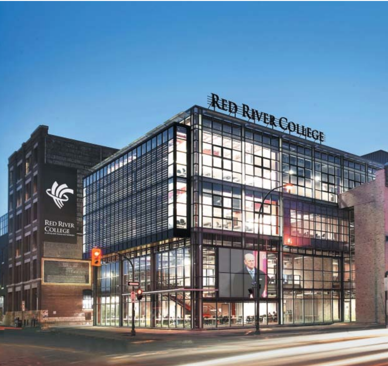
Exterior view of Red River College Princess Street Campus; Image supplied by Corbett Cibinel Architects; Copyright Gerry Kopelow
