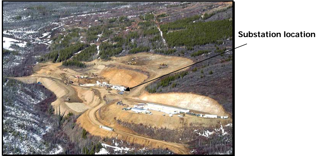
Figure 5.6-1 Location of Minto Mine Site Substation
