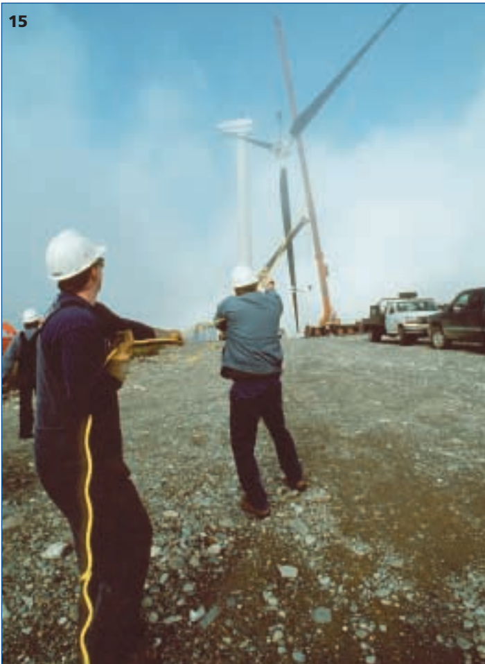
7) Hooking up the tower. 8) Setting the tower in place on its foundation. 9) Tightening one of the many bolts that holds the tower in place. 10) Looking up the ladder inside the tower. 11) Admiring the view from on high. 12) Lining up the second part of the tower. 13) Steadying the blade tip. 14) Joining a blade to the hub. 15-17) Finally, mounting the blade/hub assembly to the nacelle. 18) Congratulations on a job well done!
