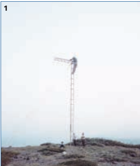
First wind monitoring tower on Haeckel Hill. 1) David Craig assembling the NRC tower. 2) Doug Craig on the ladder above the histogram recorder. 3) Gin pole used to add the third section.
