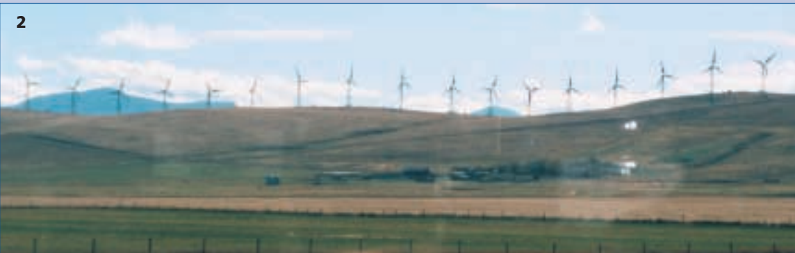
1) Pincher Creek, Alberta: vertical axis wind turbines. 2-3) Cowley Ridge, Alberta. 4) Ebeltoft, Denmark: 16 turbines service 600 homes; mid-1980s installment.
