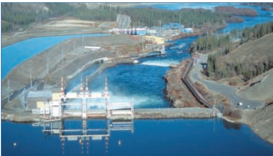
(below) Whitehorse Rapids dam. (above) One of the seven diesel generators in Whitehorse.
