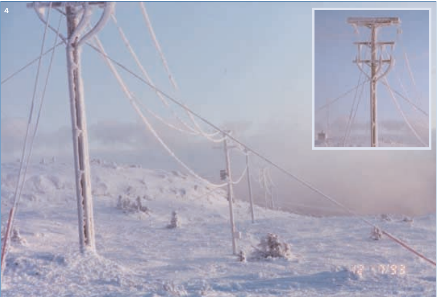
Icing on the Bonus wind turbine: 1) blade tips, 2) instrumentation, 3) blades. 4) Power lines sagging under the weight of ice. 5) Applying StaClean coating to the turbine blade. Inset photo shows heating strips.
