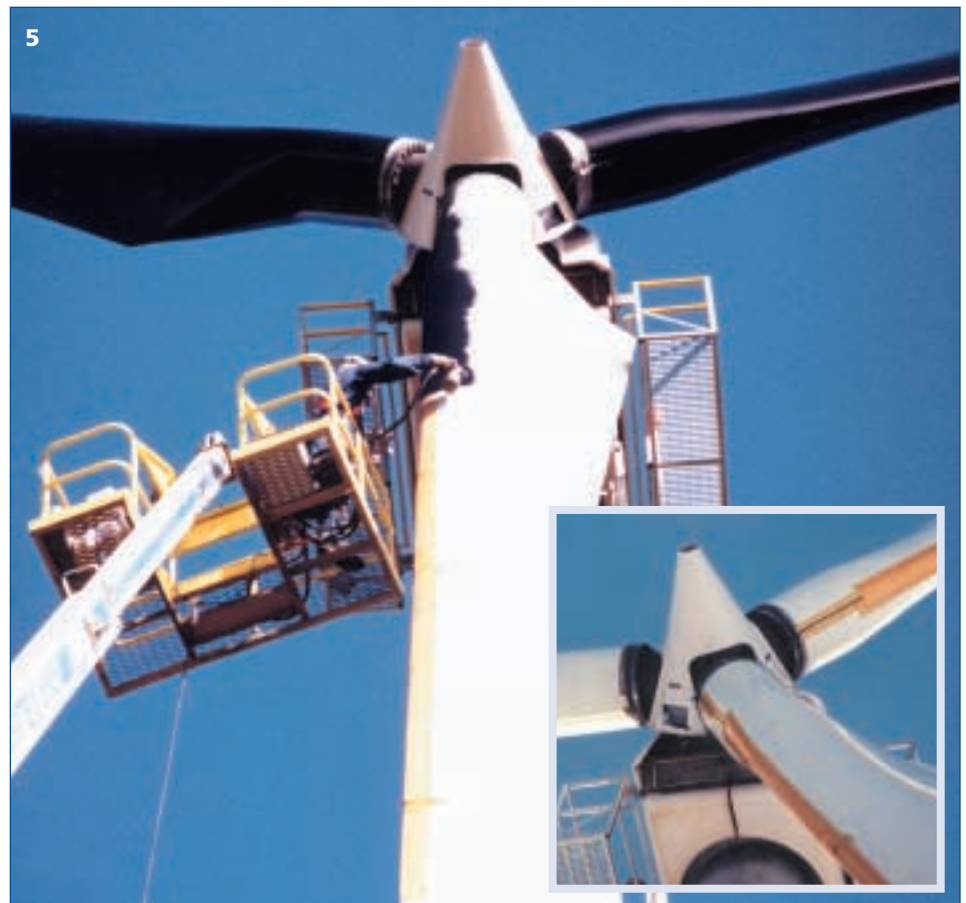
Icing on the Bonus wind turbine: 1) blade tips, 2) instrumentation, 3) blades. 4) Power lines sagging under the weight of ice. 5) Applying StaClean coating to the turbine blade. Inset photo shows heating strips.
