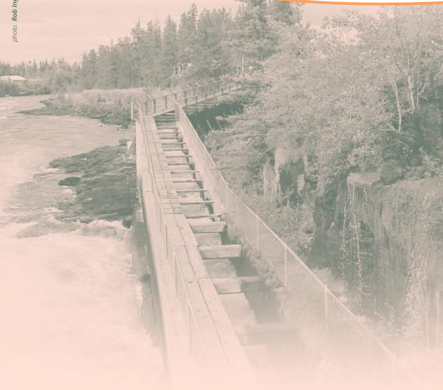
above right construction of the dam and fish ladder
