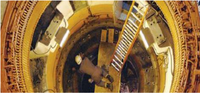
Maintenance work on one of Yukon Energy's Whitehorse Turbines ( www.archbould.com )
