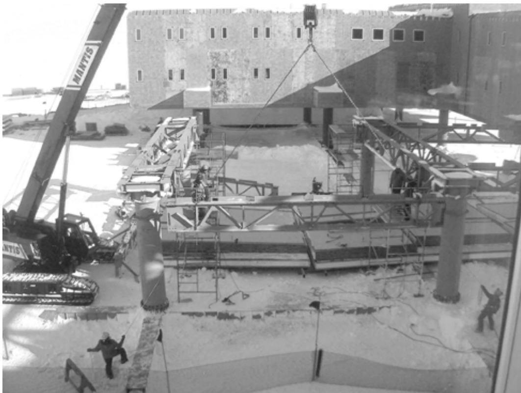
Figure 2 Workers placing steel for the A4 pod.
