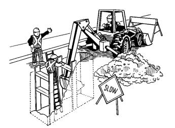
Once the worker has a minimum of two strut/ jacks placed on each set of uprights the worker may proceed to install the lower struts/jacks.
