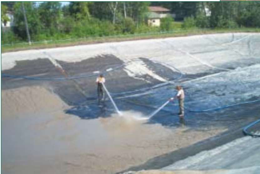
Cleaning raw water settling ponds.
