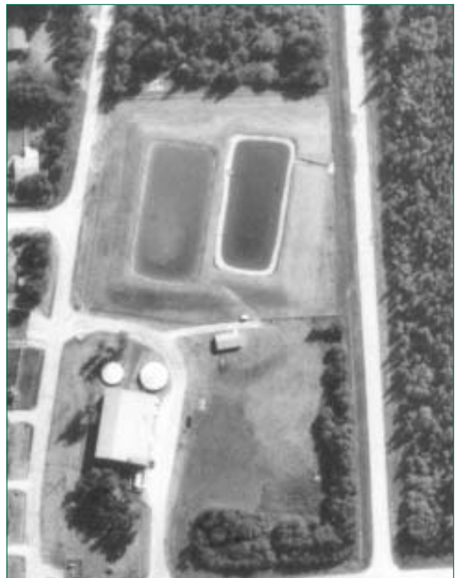
Raw water settling ponds beside water treatment plant.
