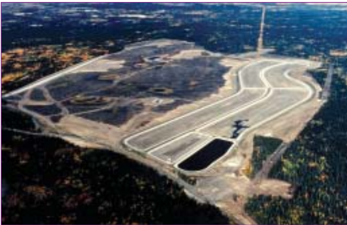
Lagoon system after construction, during initial filling.
