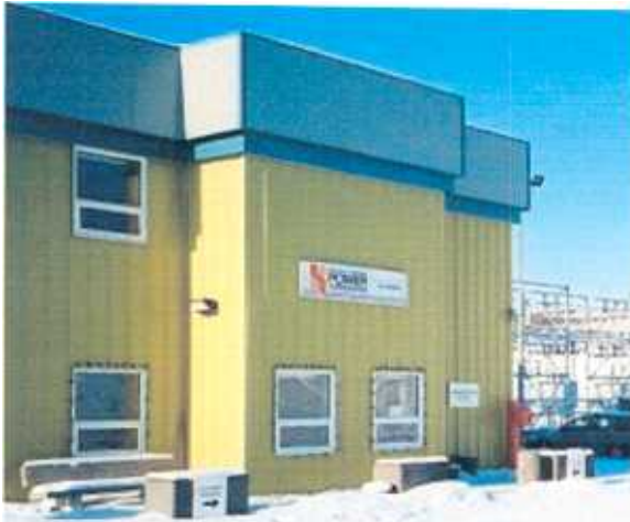
IMAGINE A PARTNERSHIP BETWEEN THE NWT POWER CORPORATION, ABORIGINAL DEVELOPMENT CORPORATIONS, AND RESOURCE DEVELOPMENT COMPANIES, TO EXPLORE HYDRO-ELECTRIC POWER GENERATION POTENTIAL.
