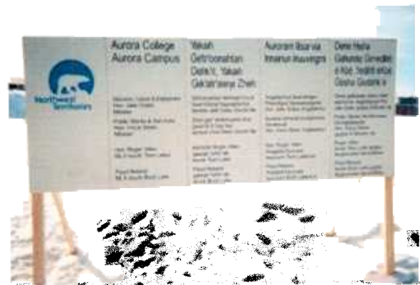
CONSTRUCTION OF THE NEW AURORA COLLEGE CAMPUS IN INUVIK WILL PROCEED AS A PARTNERSHIP BETWEEN THE GNWT, INUVIALUIT DEVELOPMENT CORPORATION, AND GWICH'IN DEVELOPMENT CORPORATION.
