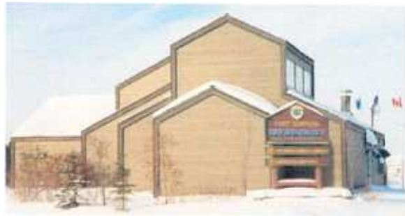
THE FORT SIMPSON VISITOR'S CENTRE HAS SUFFICIENT OFFICE AND BOARDROOM SPACE THAT IT COULD BE A MULTI-USE FACILITY FOR ORGANIZATIONS BASED IN FORT SIMPSON.
