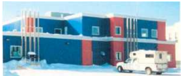
THE NEW HOSPITAL IN INUVIK WAS ORIGINALLY CONSIDERED AS A DESIGN-BUILD-FINANCE-OPERATE (DBFO) PROJECT UNDER THE P3 PILOT INITIATIVE, BUT PROCEEDED AS A DESIGN-BUILD PROJECT.
