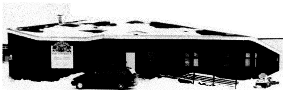
THE HAMLET OFFICE IN FORT MCPHERSON. COMMUNITY GOVERNMENTS WANT GREATER INVOLVEMENT IN THE GNWT'S CAPITAL PLANNING PROCESS. THIS COULD LEAD TO THE IDENTIFICATION OF MORE PARTNERSHIP OPPORTUNITIES.
