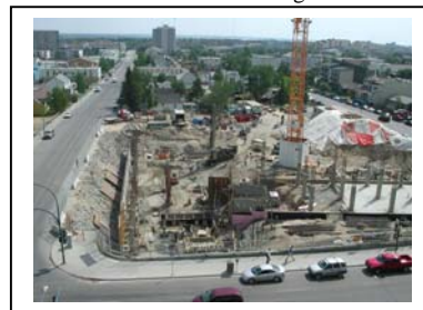
New Federal Building - 2004
