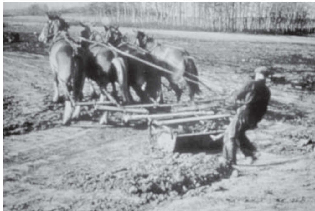
Figure 1 Horse-Drawn Excavation
