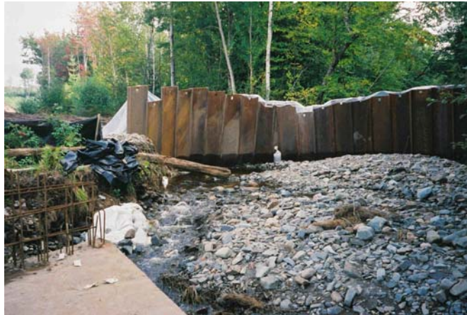
Figure 6b. Backside of the sheet pile structure following the addition of additional panels. The sand bag in center of photo indicates where the original section ended and the extended section began.
