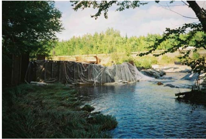
Figure 6b. Backside of the sheet pile structure following the addition of additional panels. The sand bag in center of photo indicates where the original section ended and the extended section began.
