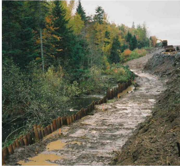
Figure 8. Retaining wall @ 16+840 showing sheet-piling barrier between construction area and Dawson Brook.
