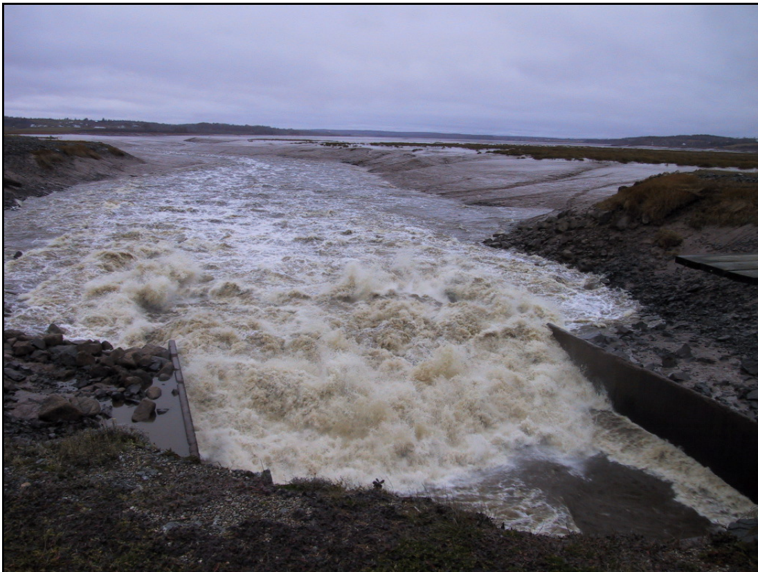
Figure 27: Freshwater discharge downstream of the Windsor tide gate following heavy rainfall in November, 2002 (photo by K. Carroll, 2002).
