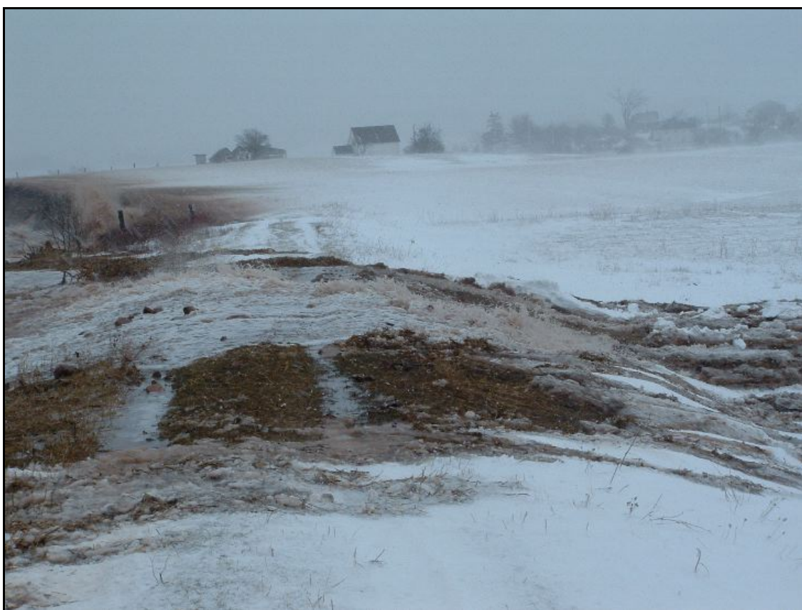
Figure 26: Storm impacts on Feb 1, 2006 at the Avonport Dyke. a) storm waves battering marsh; b) storm surge reached upper limits of dyke and c) dyke overtopped. Photo by T. Hamilton, 2006.
