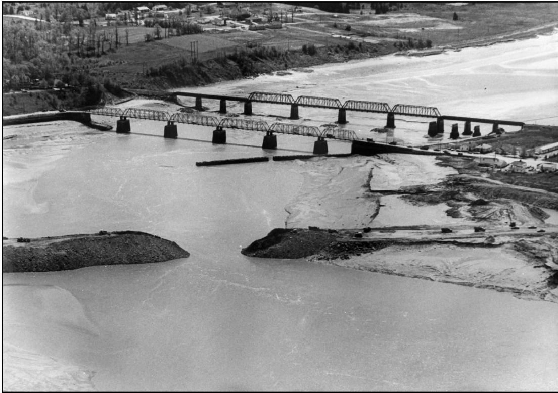
Figure 9: Final phase of the construction of the Windsor Causeway, around November, 1969. Photo from NSDA archives. Note presence of groyne installed during the construction process.
